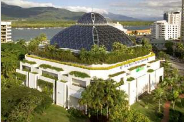
The Reef Casino architects and engineers selected a dome roof to be supported by a shell structure. Members of this shell structure were to be connected by structural nodes utilising by precision investment casting process. Precision investment casting was selected instead of sand casting so as to provide the desired form, finish, corrosion resistance and strength required for this particular architectural design application.
